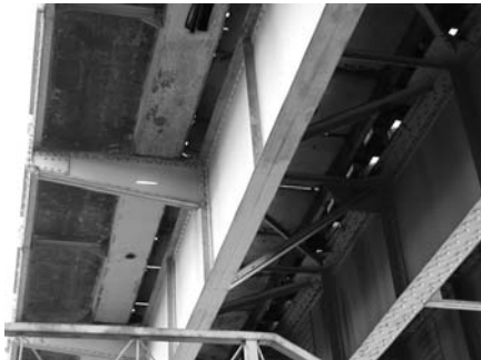
Fig. 2a: Bottom view of the bankside part of the bridge
