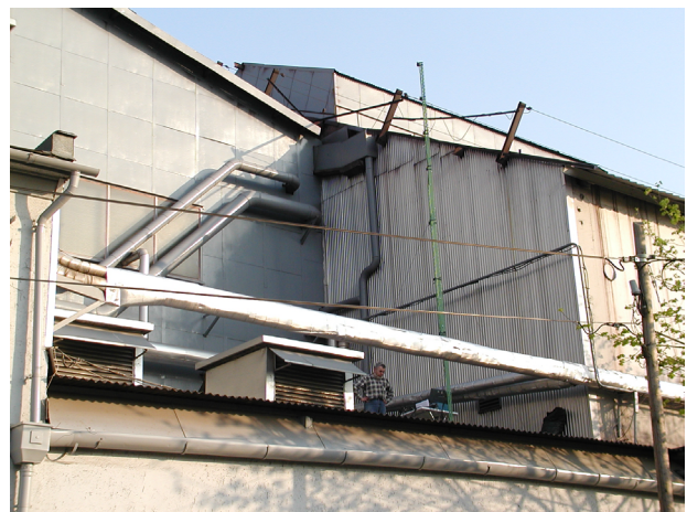
The front-side wall of the furnace bay and the bearer hall
