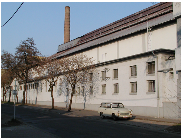
The side wall of the bearer hall
