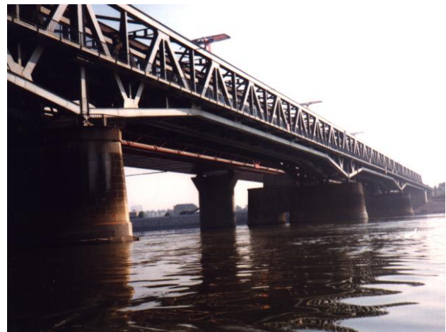
Figure 2: South rail-way bridge in Budapest above the Danube
