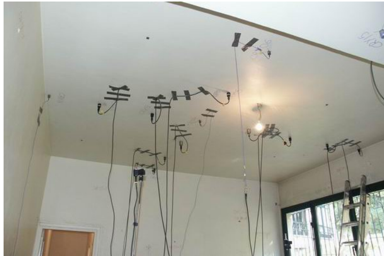
Figure 5: The measurement site in the basement with accelerometers on the ceiling
